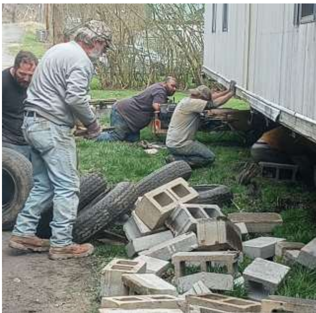
The wheels come off and the foundation blocks are set under the Packs donated mobile home
