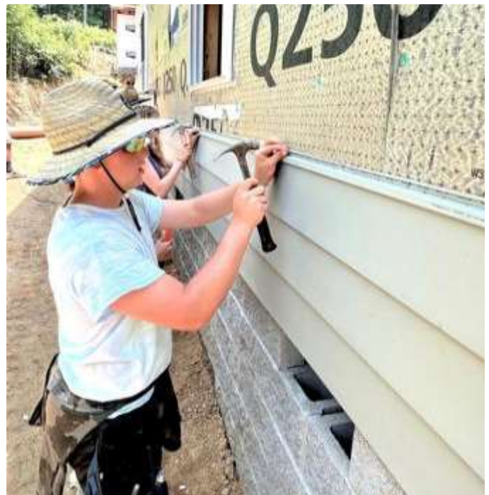
A volunteer installs siding on a local residence as part of SALS housing rehab program, photo courtesy of Beckley Register Herald
