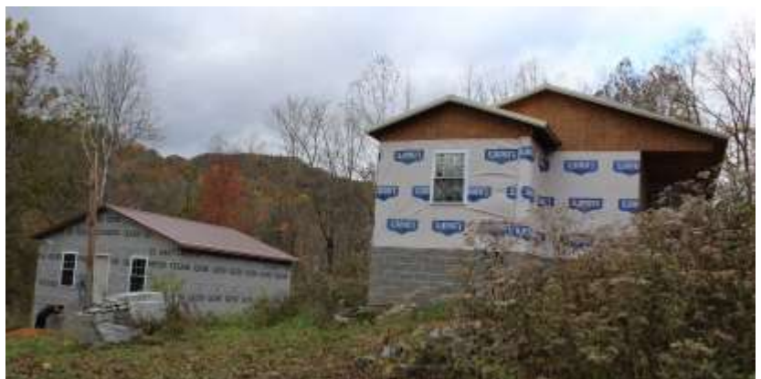
Two new affordable homes are under construction in Page WV
