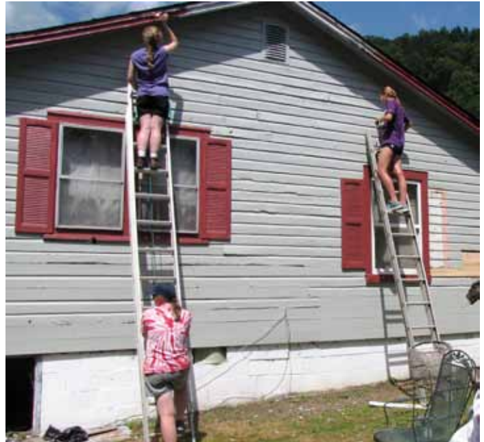
GroupWorkcamp members put new coat of paint on a home being refurbished for the residents
