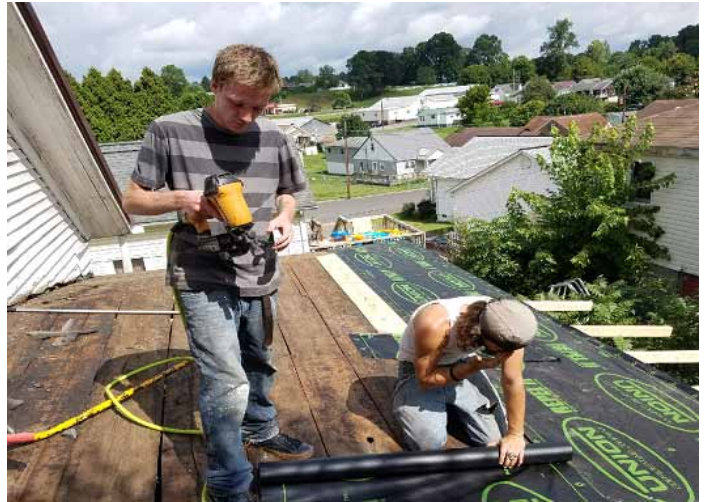
YouthBuild crew and volunteers working on replacing a roof at the Vealey home in Oak Hill.
