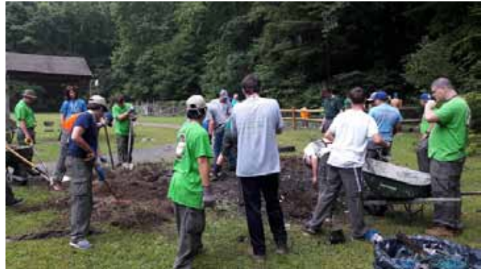
Boy Scout Jamboree volunteers make repairs at SALS
