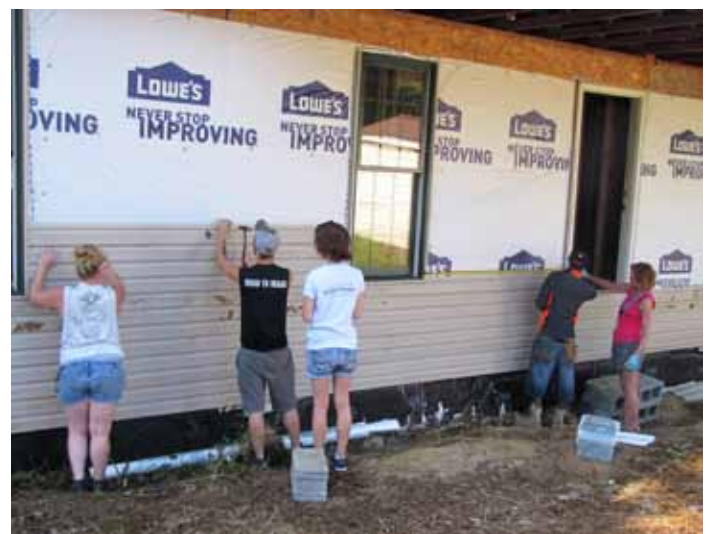
Construction crew applies siding to remodeled home
