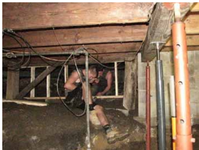
Supporting floor joists under a home in Scarboro
