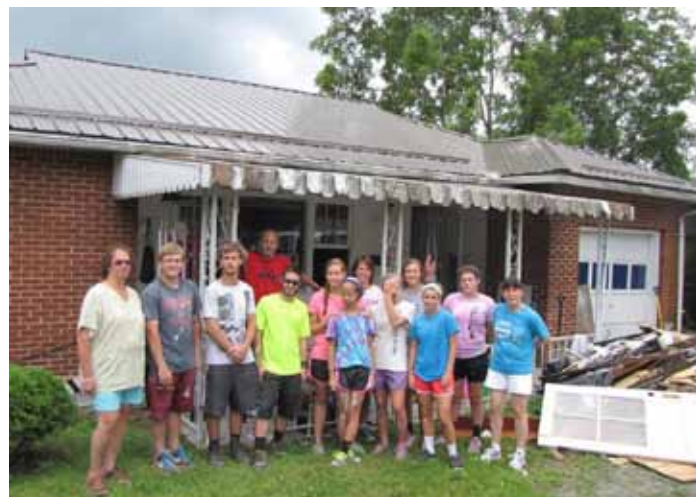
This Christian Endeavor volunteer work crew repaired roof and ceilings on the Oak Hill home of Kathy Lilly, who is pictured on the far left.
