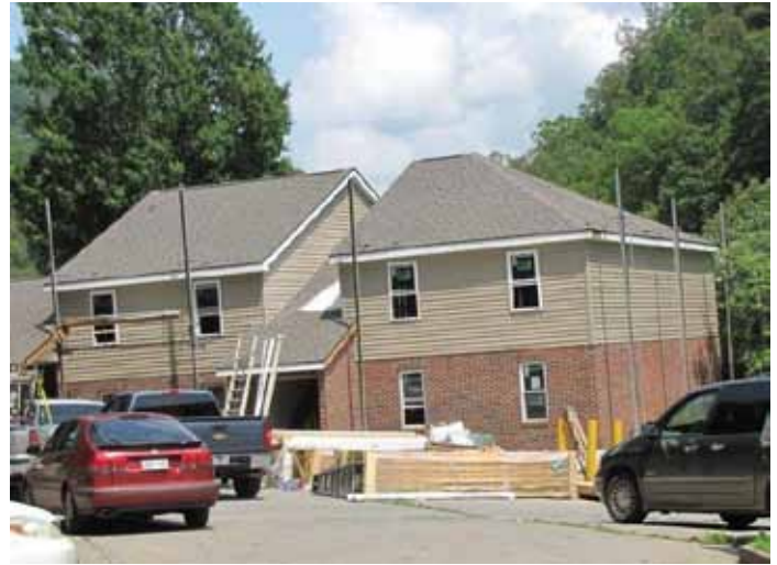
Regina Apartments SALS is building in Gauley Bridge
