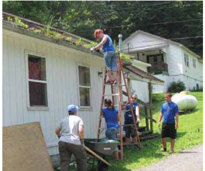
Cleaning the gutters at one of our Rehabs
