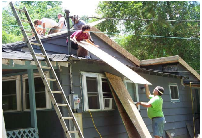
Volunteers from Christian Endeavor repair a roof
