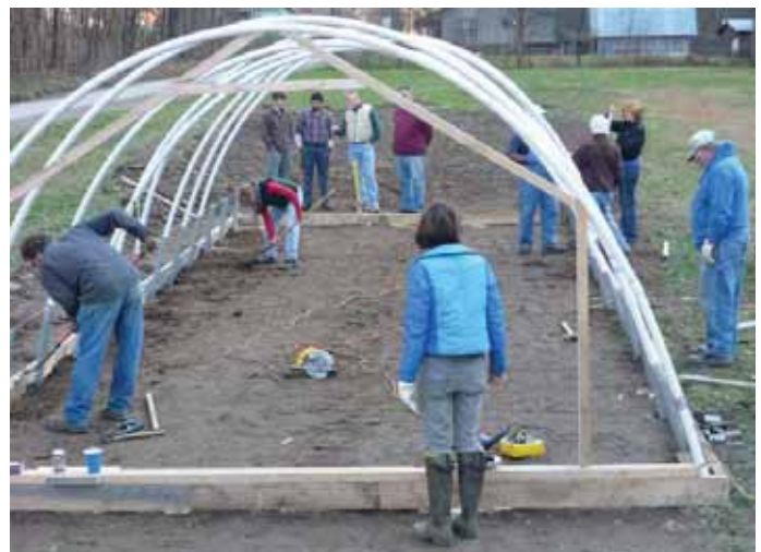
Hoop greenhouse construction at SALS
