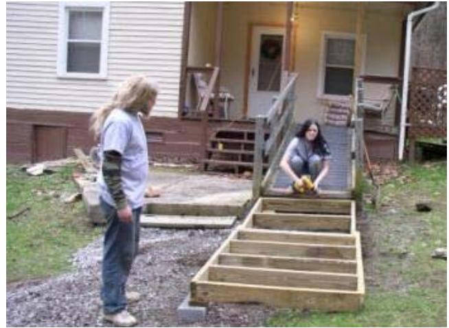
AmeriCorps members install a wheelchair ramp on home for "Make a Difference Day"
