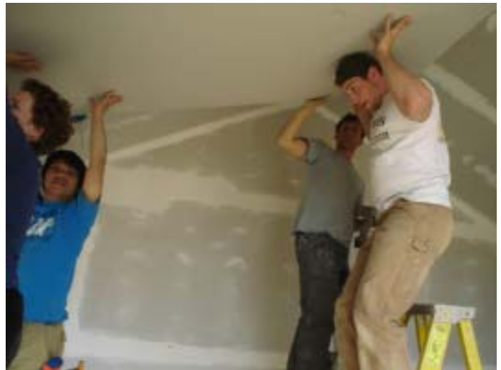
Drywall board being installed in new home at Hilltop
