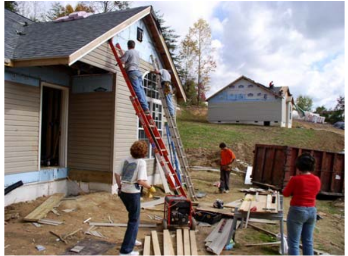
SALS crew works on new homes at Hilltop in Oakhill
