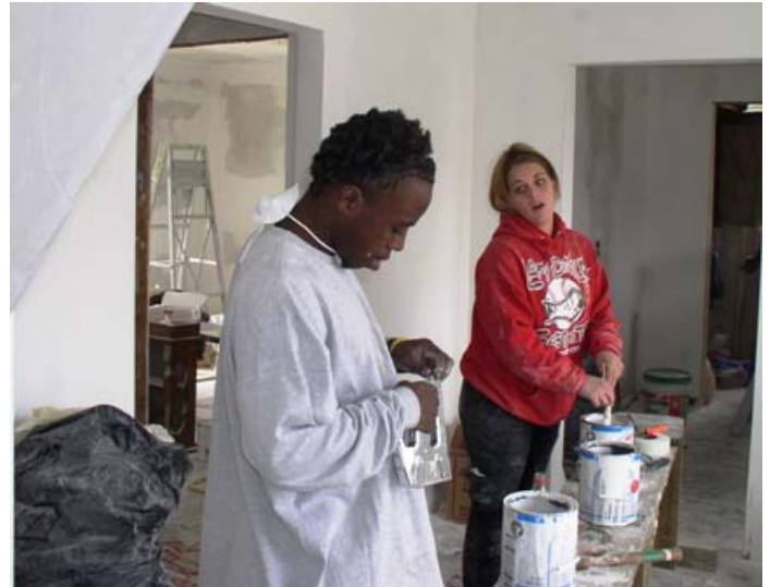
A SALS paint crew prepares to prime the walls
