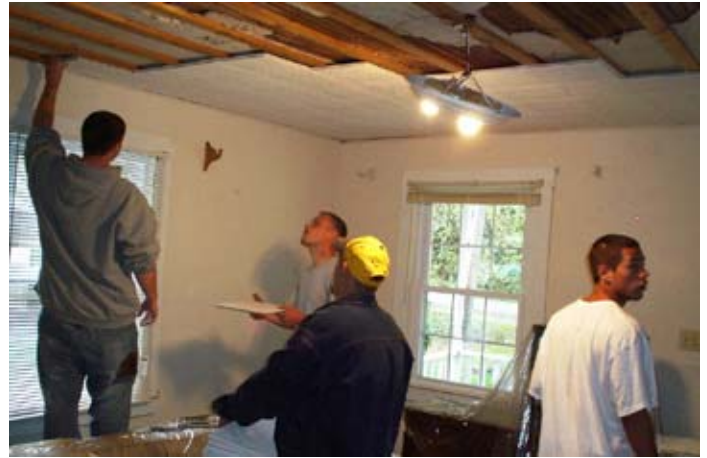
SALS crew replacing a ceiling on "Make a difference Day"
