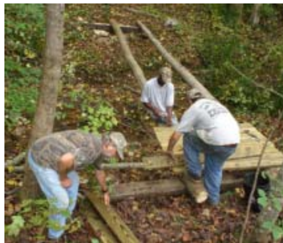
Bridge construction at SALS
