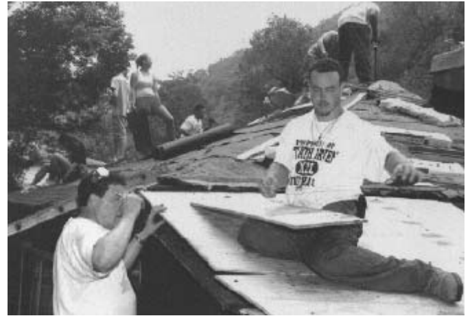
Group WorkCamps volunteers repair an old roof
