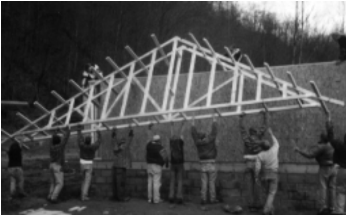
YouthBuild erects truss at New Page Housing
