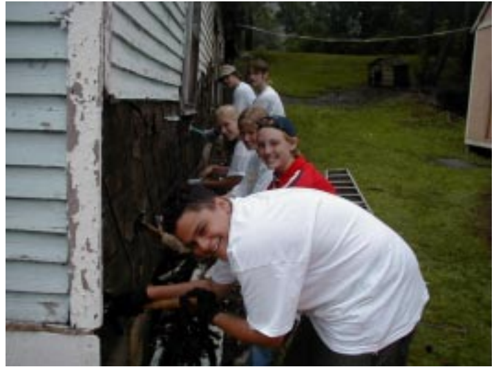
Group WorkCamp volunteers repairing home, Summer 2000
